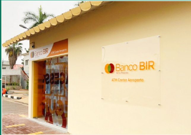
AIRPORT ATM CENTRE
